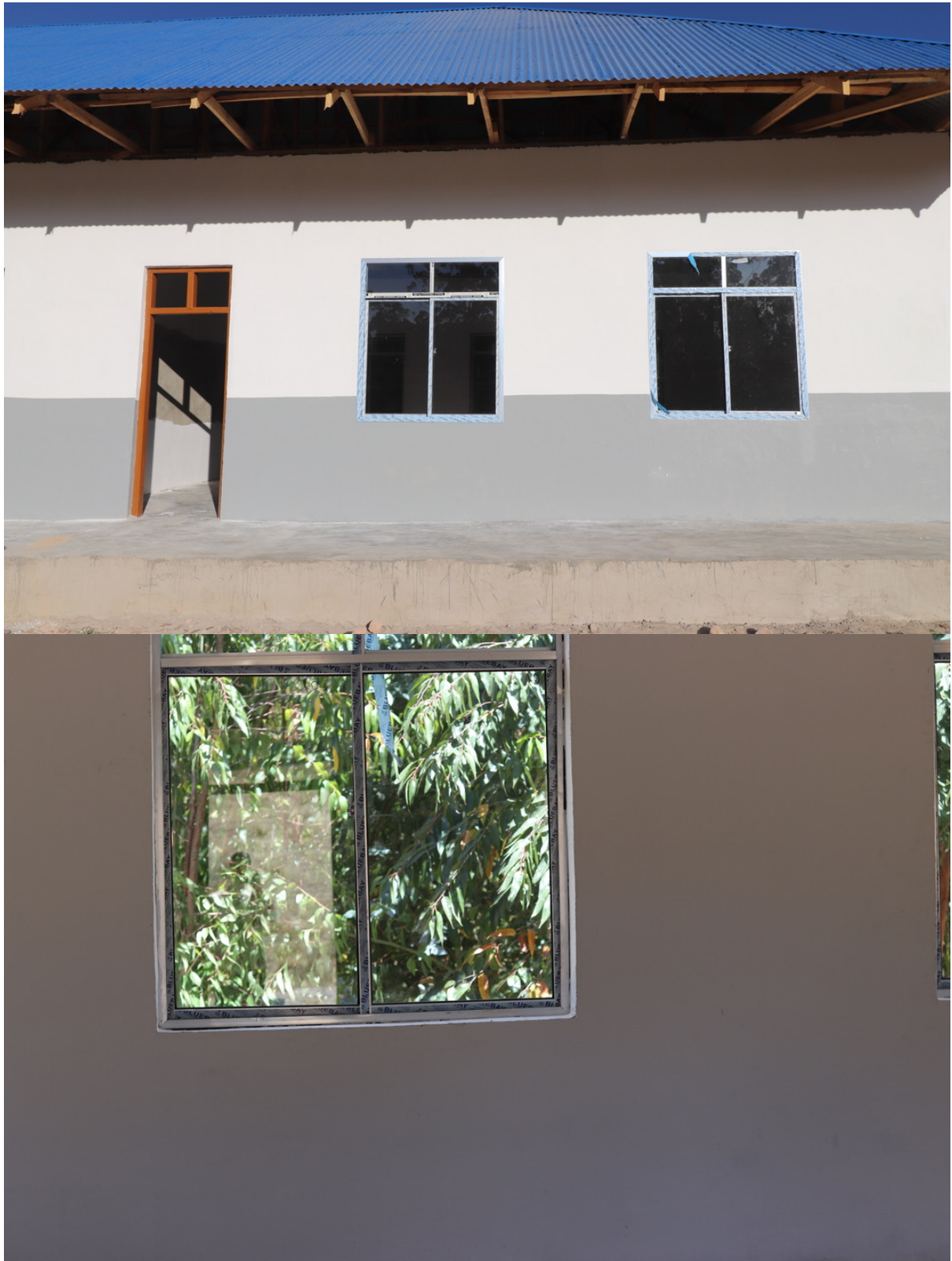
Phase 6: Installing the doors and windows (2 days of work)
